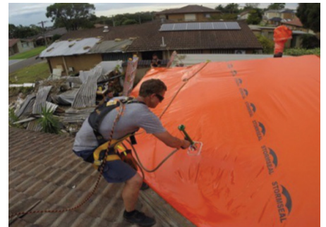
Stormseal produces a neat, tight and snug fit over a damaged roof.
